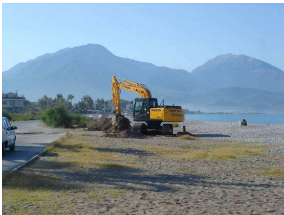
Fig 10: Excavator next to nest CS 7. Abb. 10: Bagger neben Nest CS 7.
