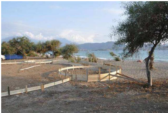
Fig.24: Wooden frame before cementation of the platform next to Bakrac, 2014.
