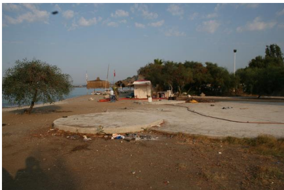
Fig.25: Completed platform near Bakrac after cementation.
