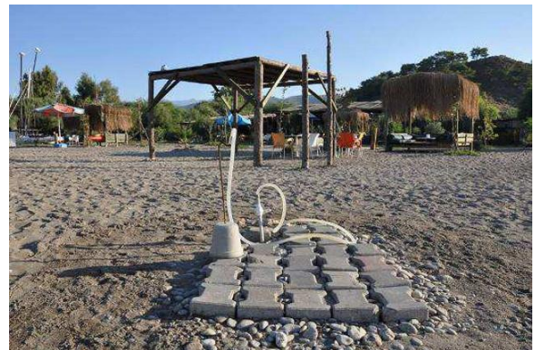
Fig.15: Wooden framework and shower platform at Spor Cafe in 2014.
