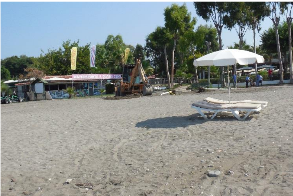
Fig. 4: Beach in front of Tuana with earth-moving vehicle at work
