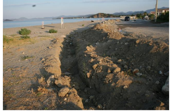
Fig.14: Re-dug trench to prevent vehicle access to beach.
