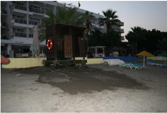
Fig.18: Showers near Aroma Beach with insufficient drainage system.
