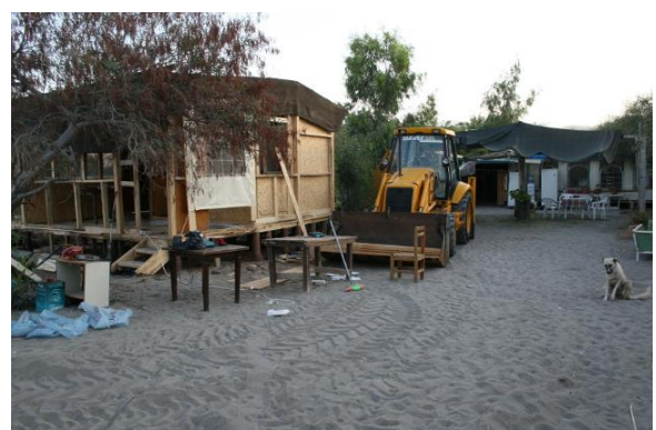
Fig.27: Recently built beach hut and heavy machinery on Çiftlik beach area.
