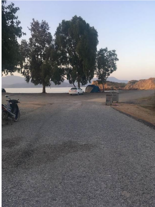
Figure 18: A newly widened and asphalted street now goes from Çalıř Beach directly to Small Beach. (Photo: M. Lambropoulos)
