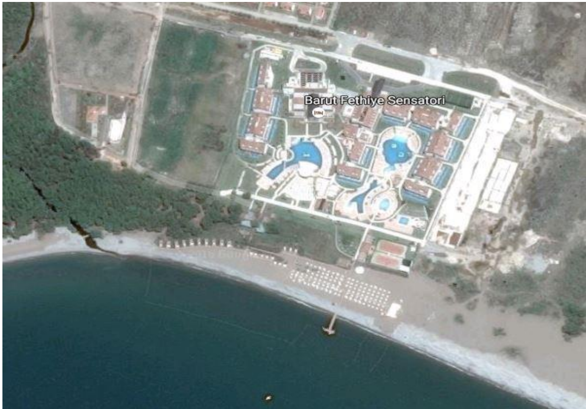
Figure 4: Aerial view of Barut Sensatori Fethiye, major parts of the beach are occupied by tourism facilities; (Photo: Google Maps, 17.10.2016)
